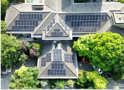
屋頂安裝分佈式光伏系統 Installation of Rooftop Distributed Photovoltaic Systems
